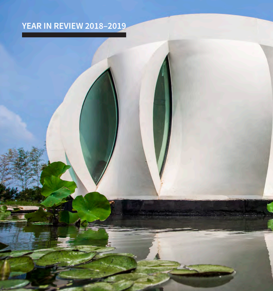
Lotus House is an energy-efficient prototype residence designed by Team WashU for Solar Decathlon China 2018.
